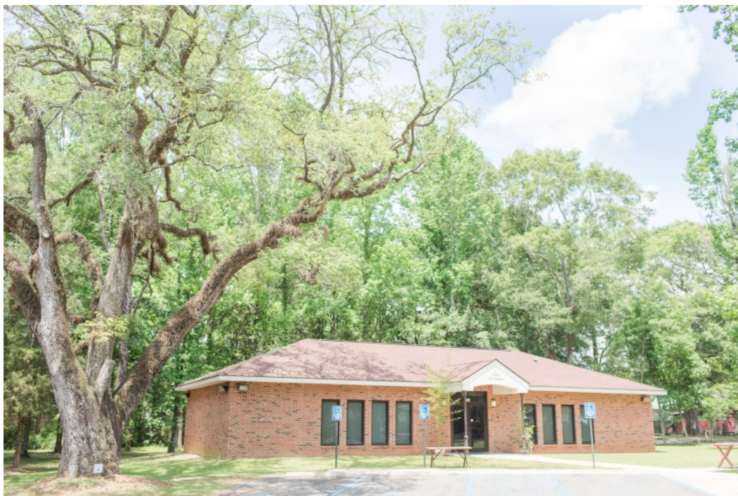
St Joseph the Worker building
